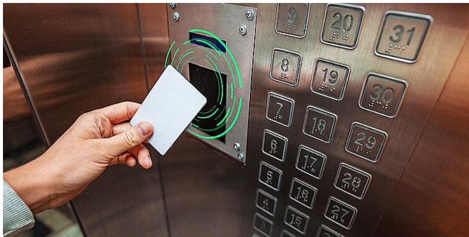
Figure 13: specific badge allowing people to reach the desired floor
